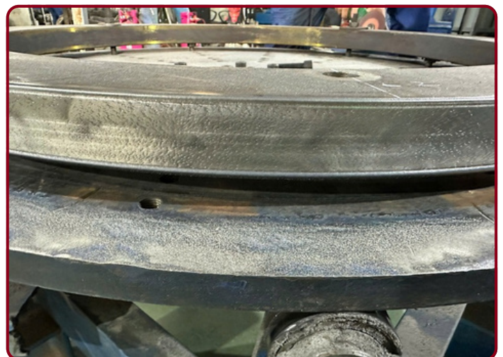
Surface After Cladding
